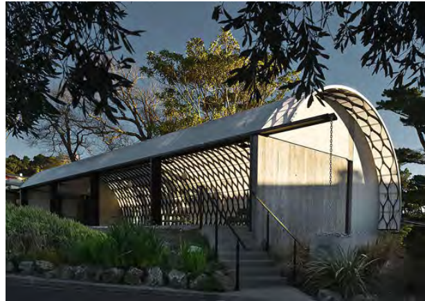
A rammed earth zoo in New Zealand by Assembly Architects Limited.
