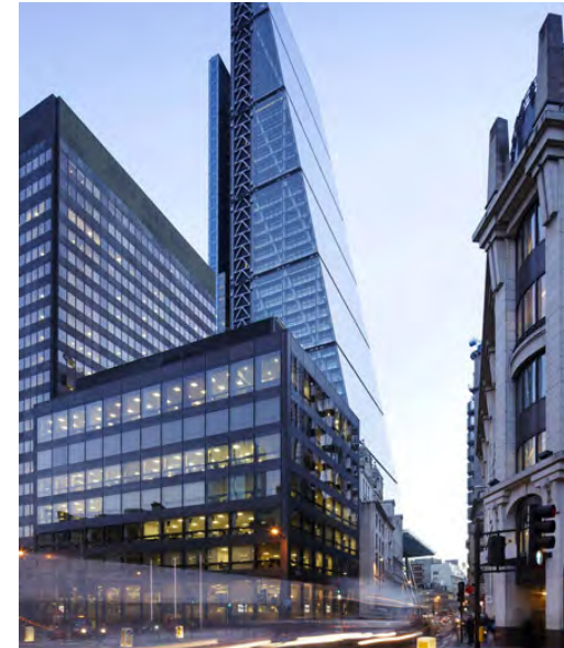
THE LEADENHALL BUILDING CITY OF LONDON
