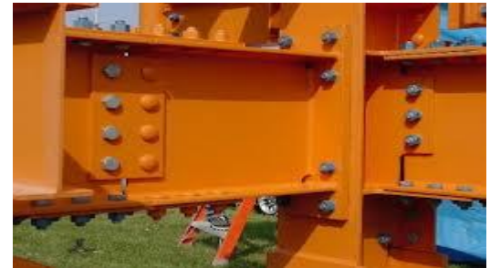
Flanged beam assemblies with the use of high-strength steel will become more compact
