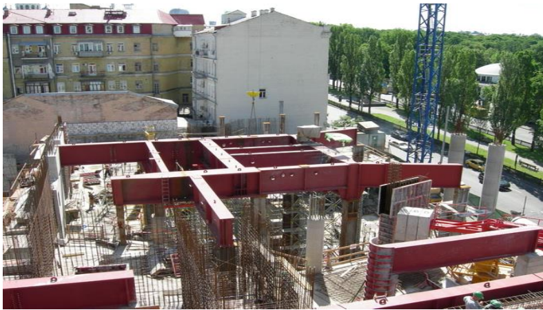
Effective solid-walled outriggers of the H-tower building 99.2 m high, made of high-strength steel 440-490 MPa. 2011
