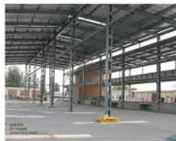
Склад CKS CENTER OF FRAME CONSTRUCTION
