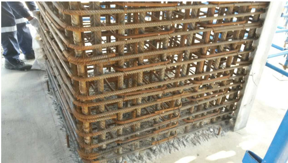
Figure 4: #3 Beam starter bars off-sets
